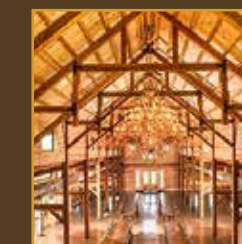
HAMMER TRUSS UPGRADE
