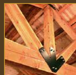
KINGPOST TRUSS UPGRADE
